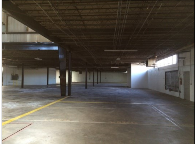
Georgia Power substation on site - sufficient electrical supply for any purpose; 100% sprinkler system throughout
